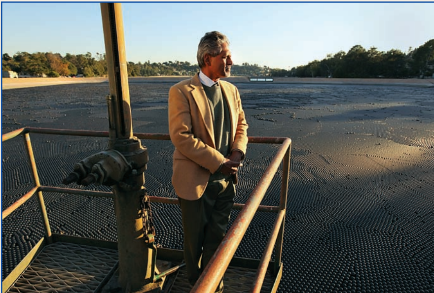
FIGURE 7.2 Dr. Pankaj Parekh, director of Water Quality for the City of Los Angeles Department of Water and Power, stands near the Ivanhoe Reservoir in Los Angeles. The reservoir is filled with black plastic balls to prevent sunlight from reaching contaminants in the water.
